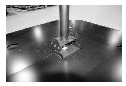
4. Following the supplied MokiTV Mount Manufacturer Installation Instructions included with your MokiTV (Part F), install the Ceiling Plate and Mast (Part B). Note: Ceiling Plate and Mast should be mounted to blocking, joist, rafter or truss that can hold a minimum of 300 lbs. DO NOT mount the MokiTV directly into drywall.
